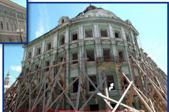
Kazan Hotel in the Baumann Street
