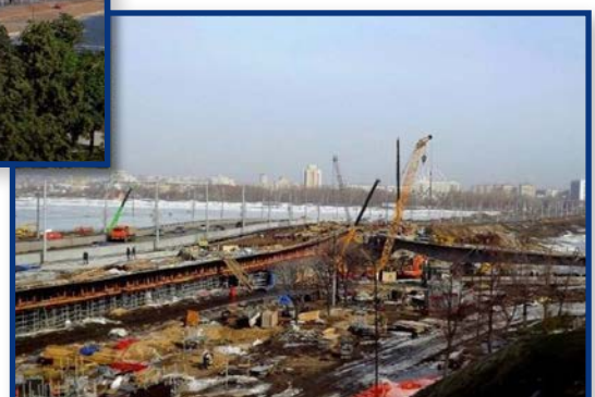
Leninskaya Dam Reconstruction
